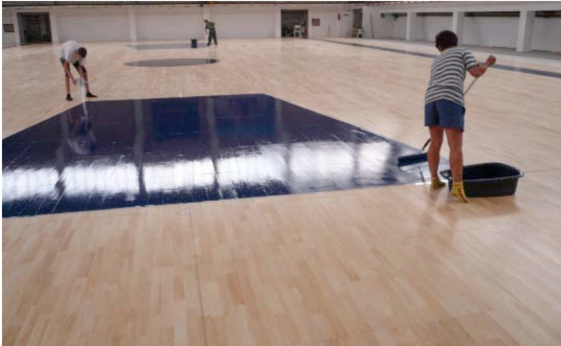
Once all the 1,100 panels had been laid, the court was marked for play.
