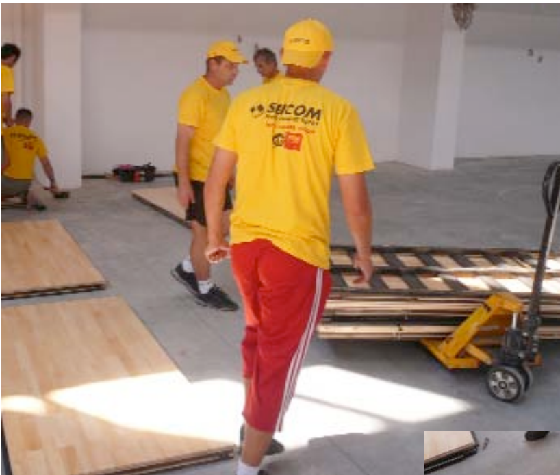
The first phases in the laying of the removable 22 mm wood parquet panels.
