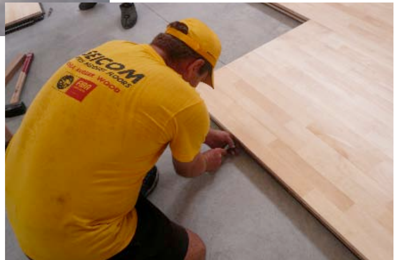
After laying, all the panels require is locking with the special key provided.
